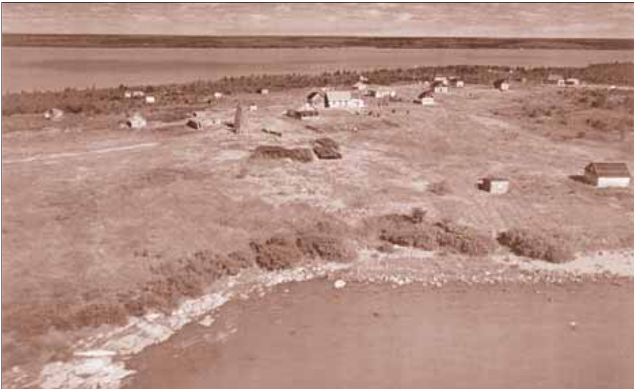
Early Split Lake settlement in 1925 showing Hudson's Bay Company buildings and residences.
