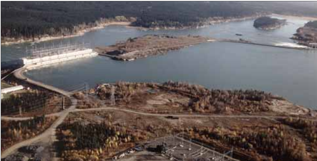
Kelsey dam and generating station located on the Nelson River where it flows into Split Lake. Construction began in 1956 and the first four turbines started operating in 1960.
